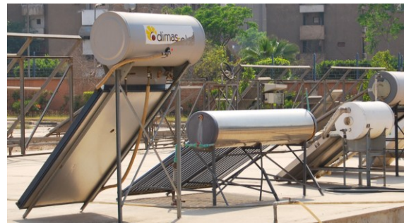
Flatplate & evacuated tube SWHs (thermosyphon)
