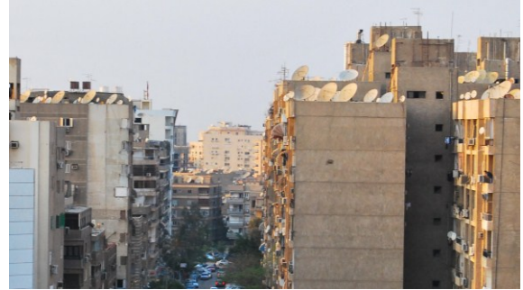
Current building design with satellite dishes
